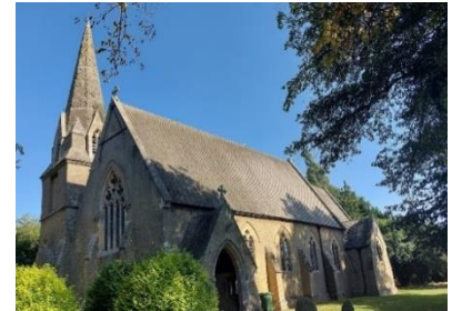
St Mark's, Friday Bridge
