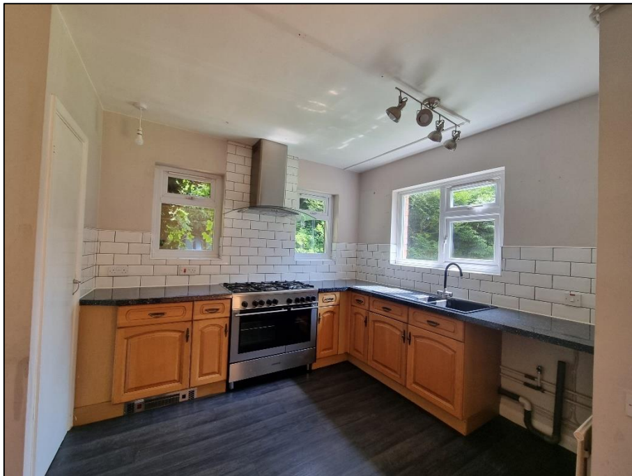
The Kitchen is Part Tiled and in Good Order
