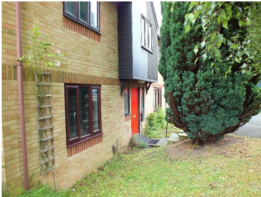
Figure 17 – Vicarage main entrance
